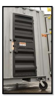
door entries. Both doors are equipped with two brackets for sliding a 1 in. x 1 in. wooden piece across, increasing the difficulty of entry.
