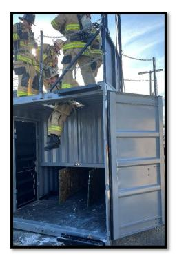
Confined Space: Positioned under the adjustable pitched roof, the confined space comes standard with four pieces of Unistrut to create two OSB walls. The Unistrut is bolted to the ground and to the ceiling which can be easily moved with a drill. The confined space section was designed to have endless iterations to keep trainees from getting used to the configuration. The front of the confined space has slides which
