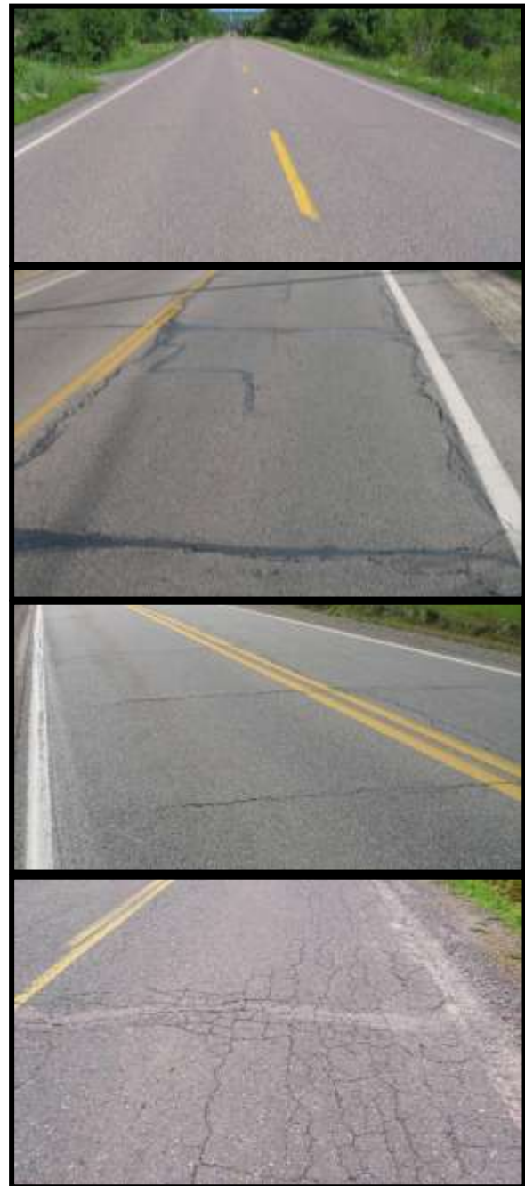
Figure 2: Top image – PASER 8 road that is considered “Good” by the TAMC exhibit only minor defects. Second image – PASER 5 road that is considered “Fair” by the TAMC. Exhibiting structural soundness but could benefit from CPM. Third image – PASER 6 road that is considered “Fair” by the TAMC. Bottom image – PASER 2 road that is considered “Poor” by the TAMC exhibiting significant structural distress.
