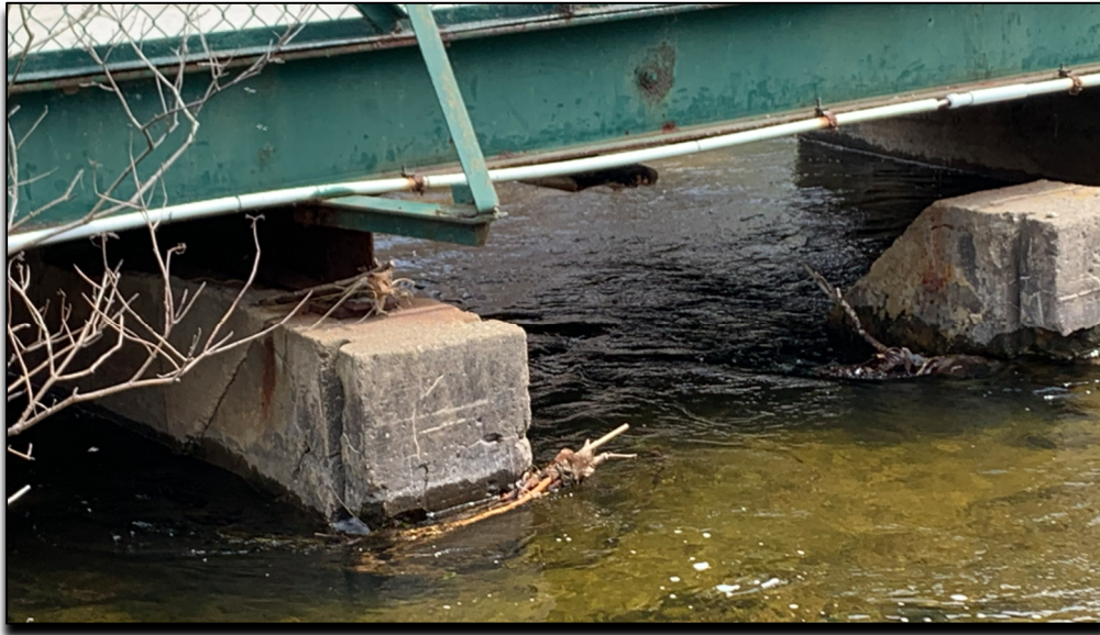
Image 1 – Existing bridge mid-span supports
