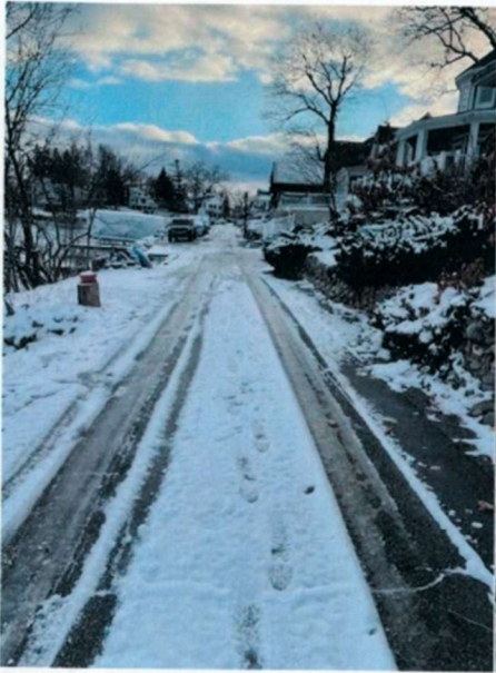
Longpointe Drive Thursday 12/5/2024 no Snowplowing called Village
