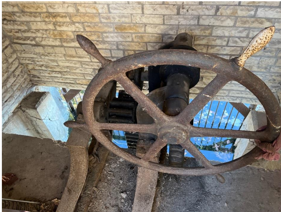
Photo #18: Auxiliary Spillway Gate.
