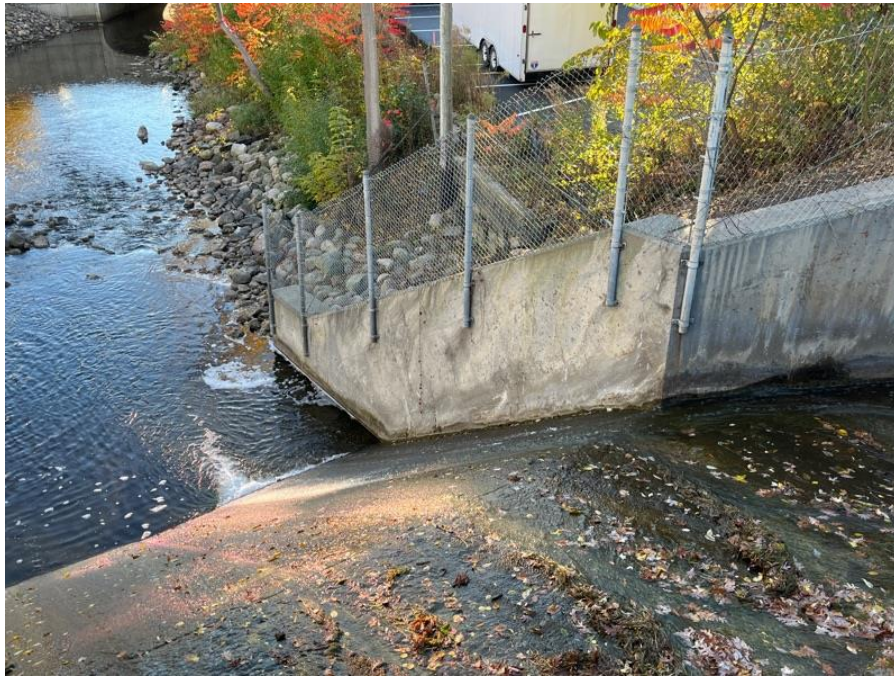
Photo #11: Principal Spillway Abutment Right Wall.
