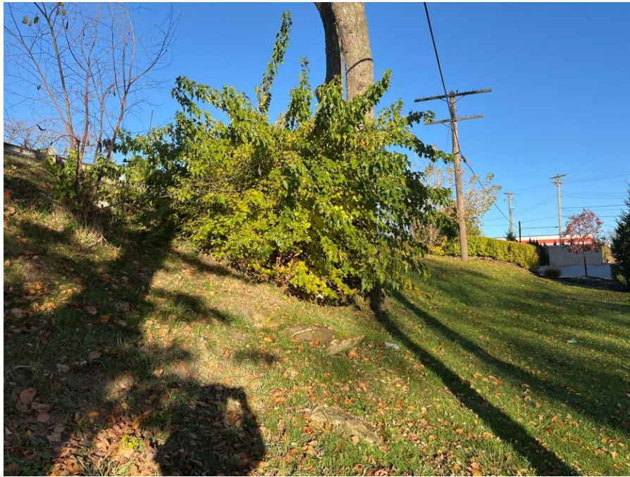
Photo #37: Embankment Downstream Slope. Left slope shown. Issue: Trees and Brush, Action: Maintenance
