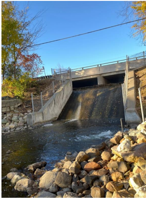
Photo #3: Principal Spillway Weir Wall.
