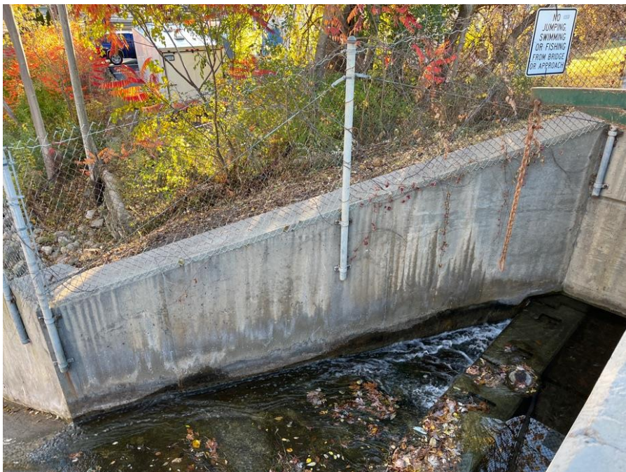
Photo #10: Principal Spillway Abutment Right Wall.
