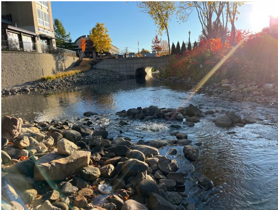
Photo #12: Principal Spillway Apron. Receiving channel.
