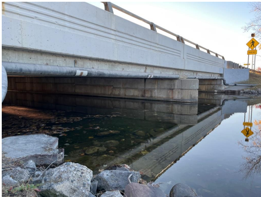
Photo #4: Principal Spillway Inlet.
