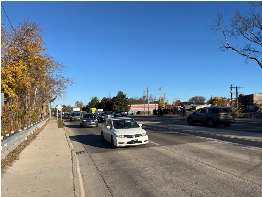
Photo #32: Embankment Crest. Crest is M-24, viewed from right.
