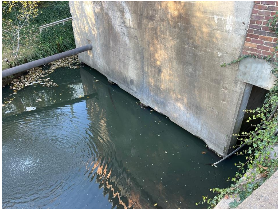
Photo #16: Auxiliary Spillway Outlet Conduit.
