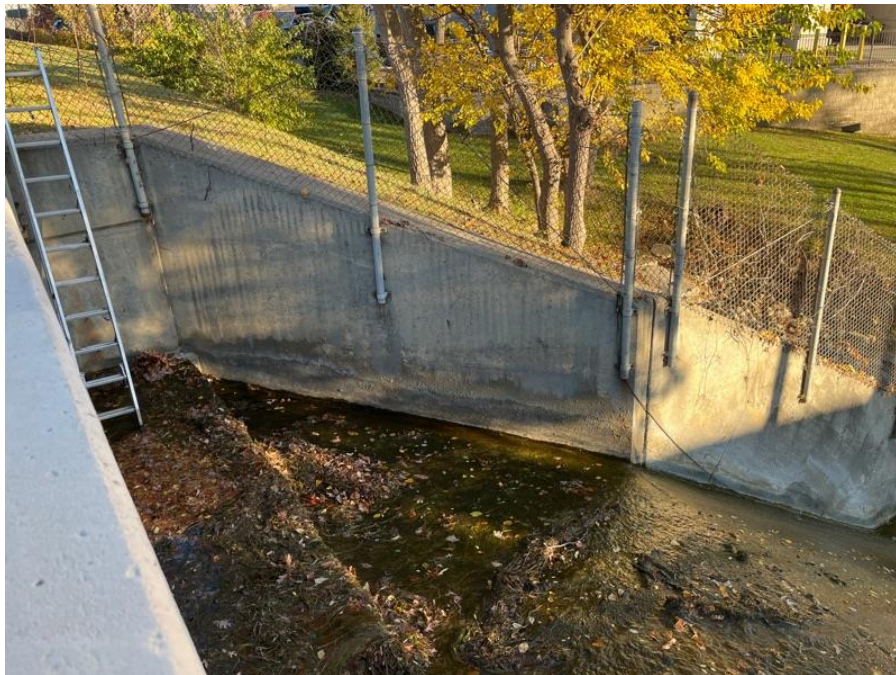
Photo #8: Principal Spillway Abutment Left Wall.
