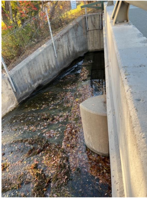
Photo #1: Principal Spillway Weir Wall. Concrete block stoplogs shown.
