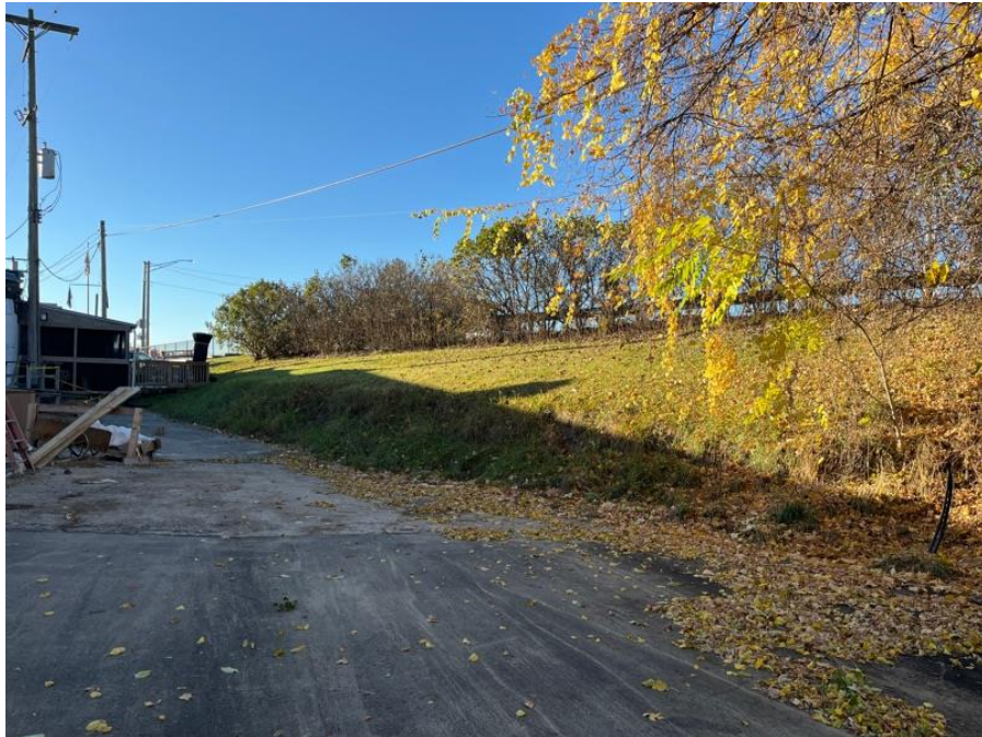
Photo #40: Embankment Downstream Slope. Right slope shown.
