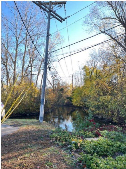
Photo #17: Auxiliary Spillway Outlet Conduit. Principal spillway receiving channel (shown on left side of photo) and auxiliary spillway channel rejoin to Paint Creek.
