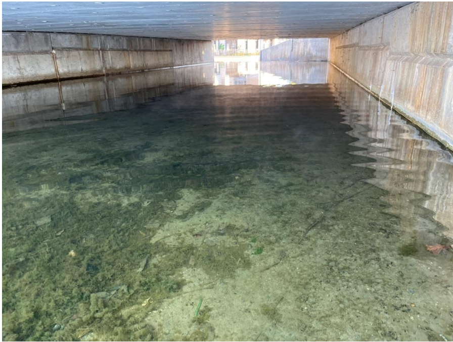
Photo #7: Principal Spillway Inlet.
