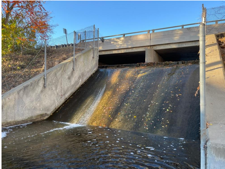
Photo #2: Principal Spillway Weir Wall.
