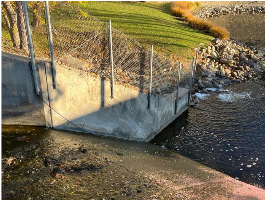
Photo #9: Principal Spillway Abutment Left Wall.
