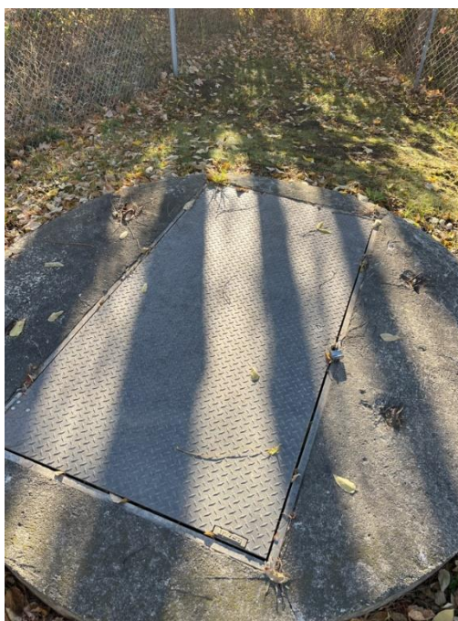
Photo #26: Embankment Upstream Slope. Cold water inlet at the park immediately north of the dam.
