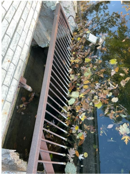
Photo #19: Auxiliary Spillway Gate. Upstream face.
