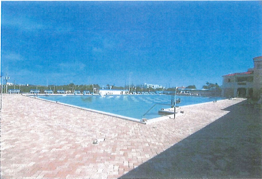
EXHIBIT 1. OVERALL VIEW OF POOL AND DECK LOOKING NORTHWEST
