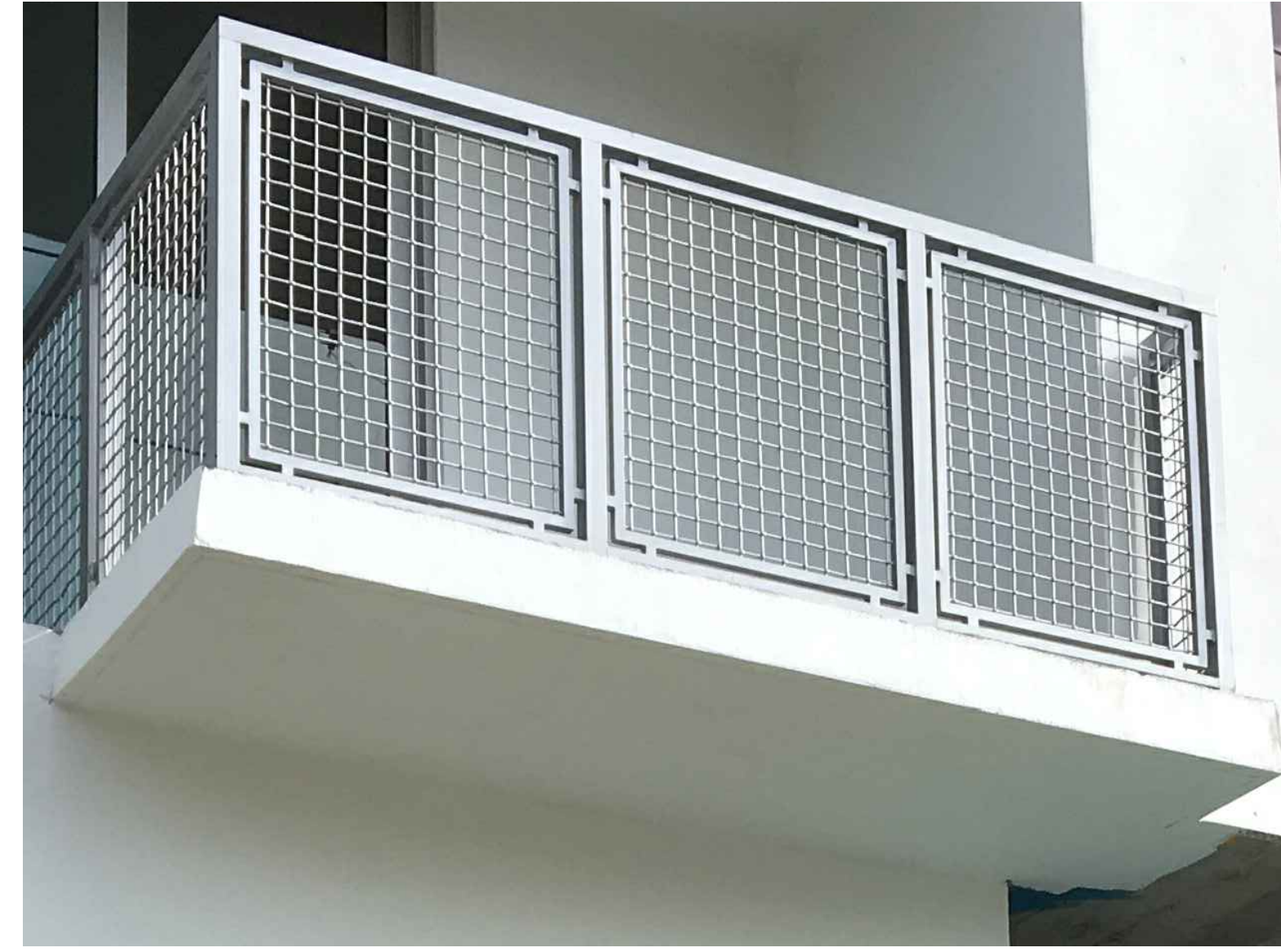
3 PERFORATED METAL MESH RAILING
