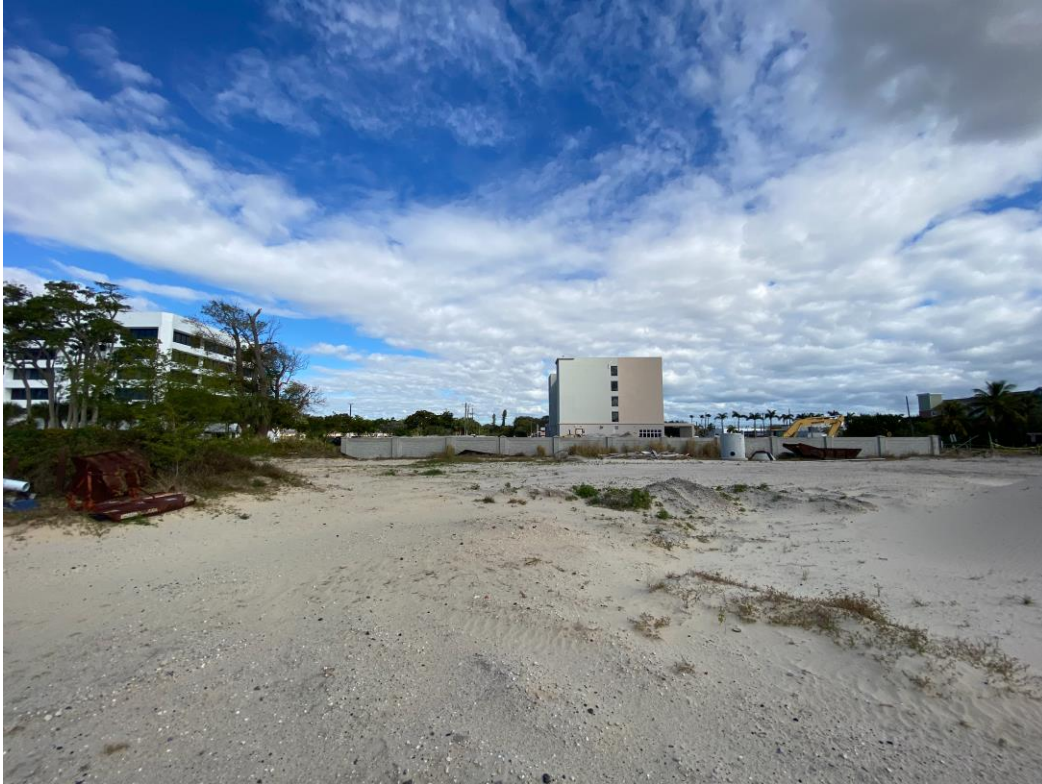
NORTH – ADJACENT SURROUDNING SITE
