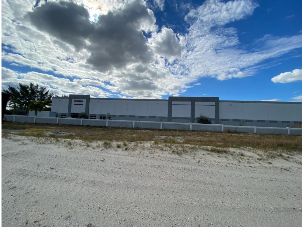
SOUTH – ADJACENT SOURROUNDING SITE
