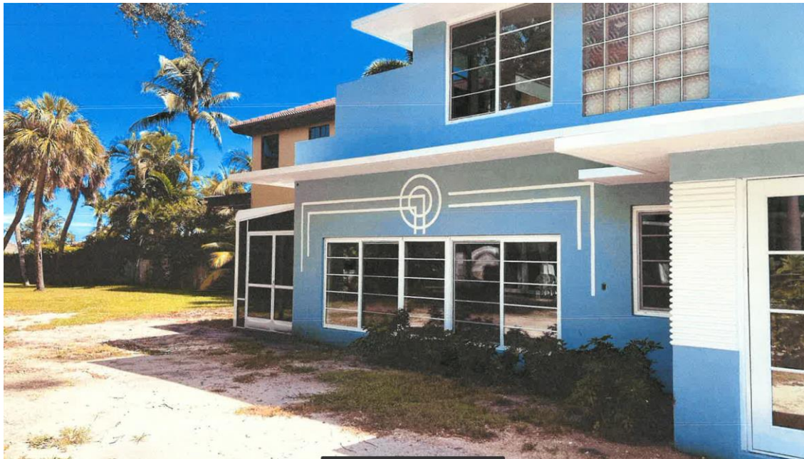
Proposed Carport Demolition:
