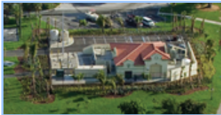
Regional Sewer pipelining & Replacement system
