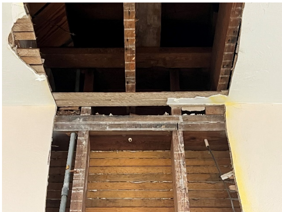
Photo 3. Floor joist bearing on the wood framed wall
