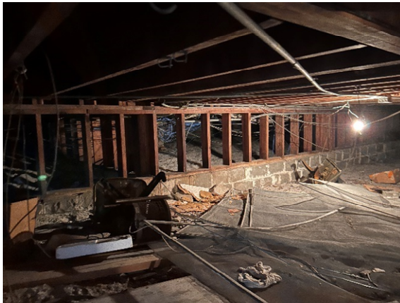
Photo 1. Floor joist bearing on Wood Stem wall at the crawl space
