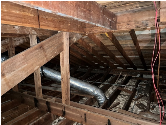
Photo 4. Roof framing view from attic space
