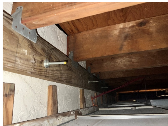
Photo 2. Floor joist to exterior CMU wall
