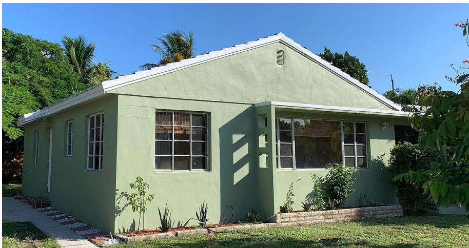
Existing Flat Concrete Tile Roof
