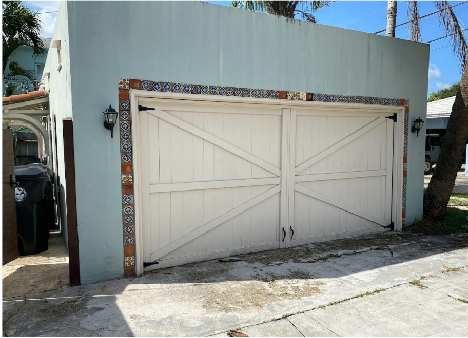
Existing carriage style garage door.
