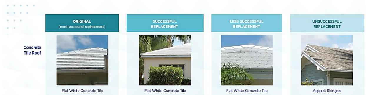
Roof material is an important character-defining feature for a historic property. Per the Design Guidelines, new flat white concrete tiles are the only successful replacement options for original flat white tile roofs. Flat white concrete tiles that replicate historic tile profiles and dimensions are still in production today, and could be utilized as the replacement roofing material.
