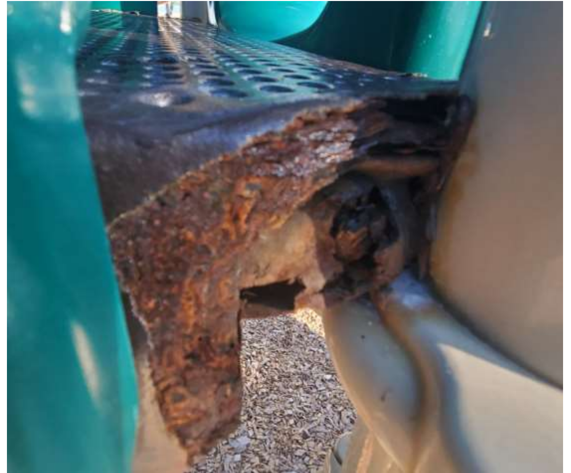
Fig 4.2 Corrosion of platform number 1
