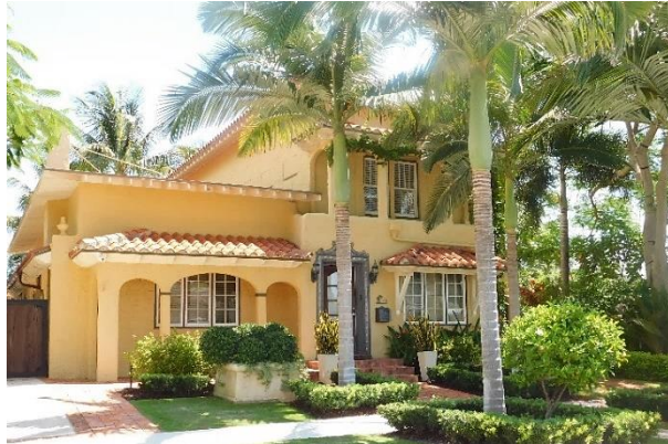
Example: 162 Auburn Drive Original Wood Double-Hung and Casement Windows
