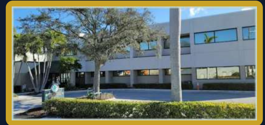
PBSO District 14 Substation
