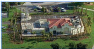
Regional Sewer pipelining & Replacement system
