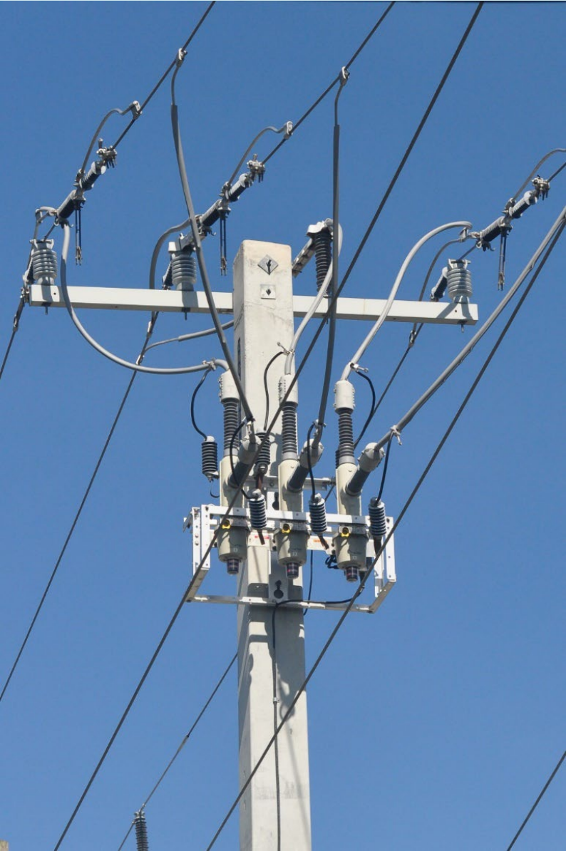
Mid-point Reclosers – smaller circuits
