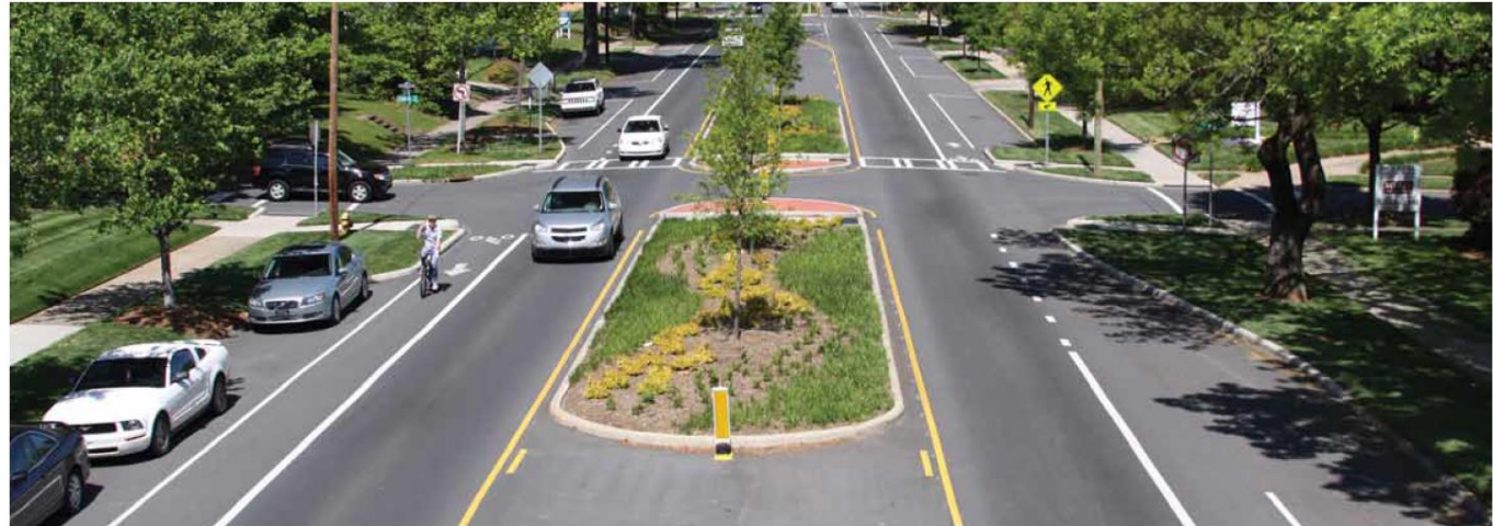
In addition to making East Boulevard in Charlotte, N.C., more attractive, a road diet reduced travel speeds, bicycle and pedestrian injury rates and the number of rear-end and left-turn collisions. Photo courtesy city of Charlotte
