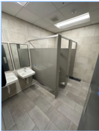
Firestation Bathroom Remodel.jpg
