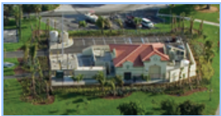
Regional Sewer pipelining & Replacement system
