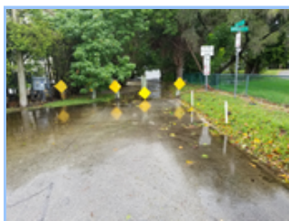
Stormwater Collection and Conveyance
