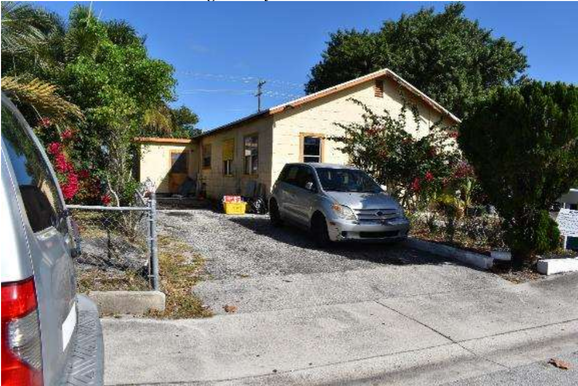
View looking southeasterly of 706 South H Street
