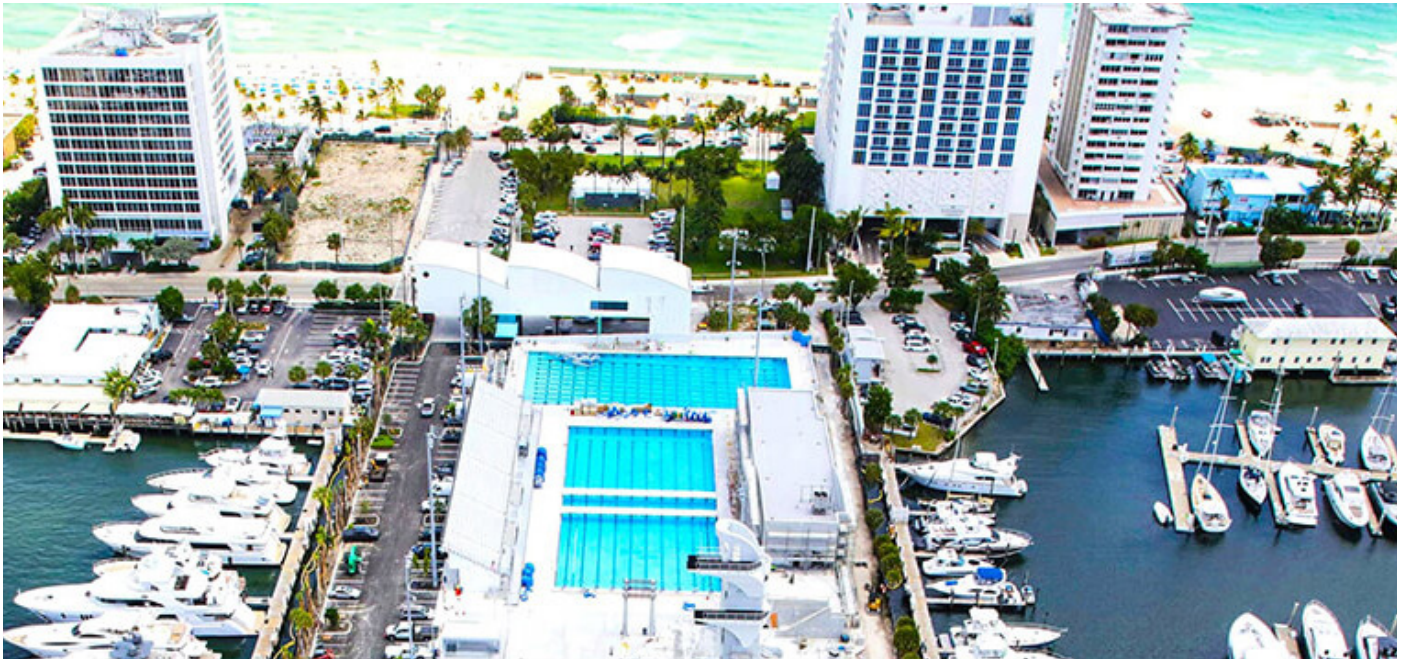
FORT LAUDERDALE AQUATIC COMPLEX PROJECT COMPLETED BY SRS, A WHOLLY OWNED SUBSIDIARY OF ZYSCOVICH
