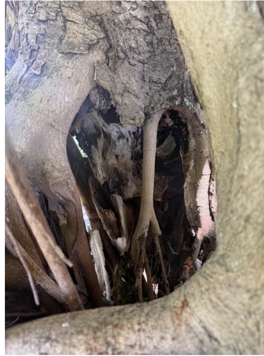
Fig. 7 Interior cavity — degraded wood and open voids within the stem.
