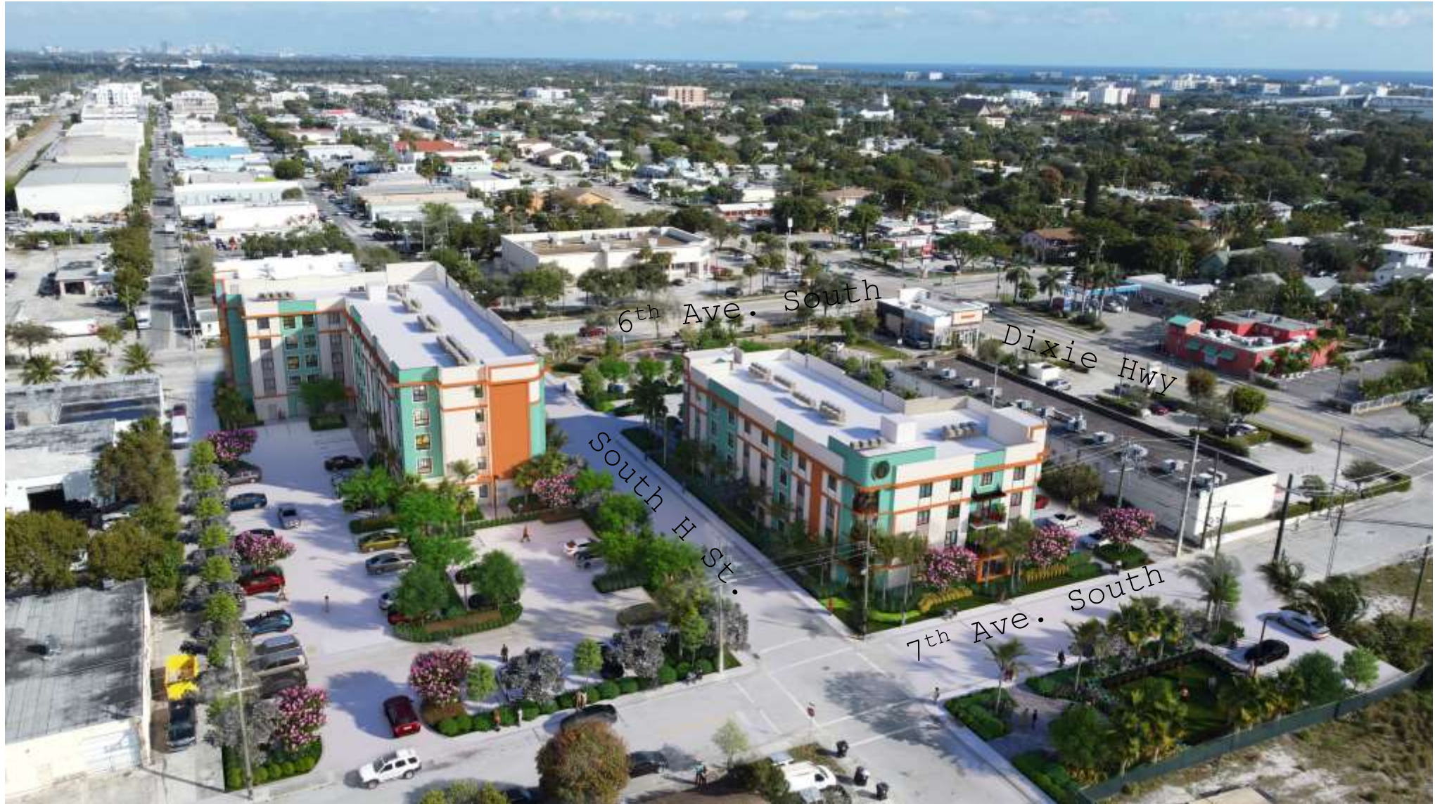
Aerial – Looking Northeast
