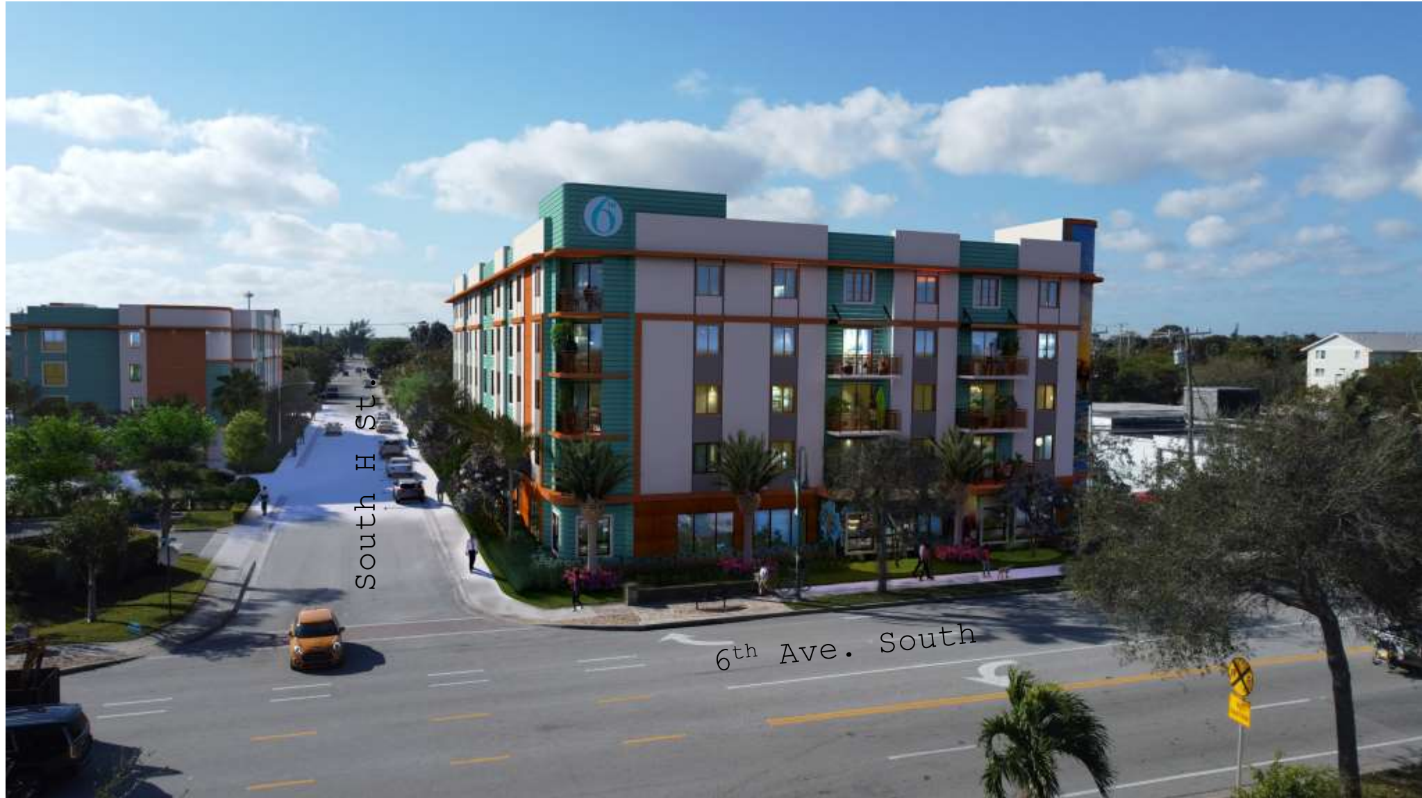
Aerial – Building A looking South
