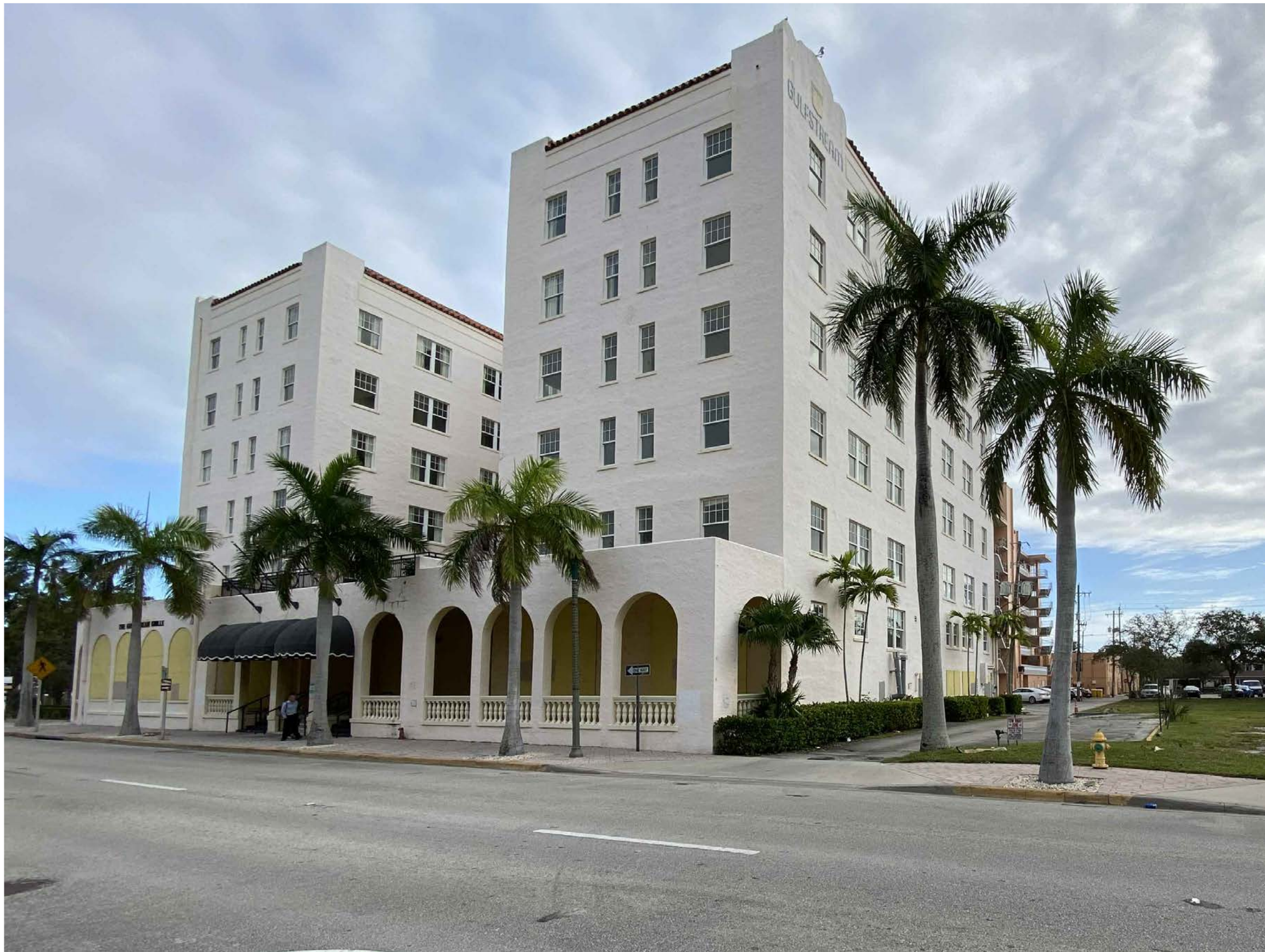
EXISTING BUILDING LOOKING SOUTHEAST ARCADE, DECORATIVE PARAPET, TRIMS, RAILINGS, TILE ROOF, SHIELDS AND SIGNAGE TO REMAIN. EXISTING WINDOWS AND DOORS TO BE REPLACED WITH NEW WINDOWS AND DOORS (MULLION CONFIGURATION TO MATCH EXISTING)
