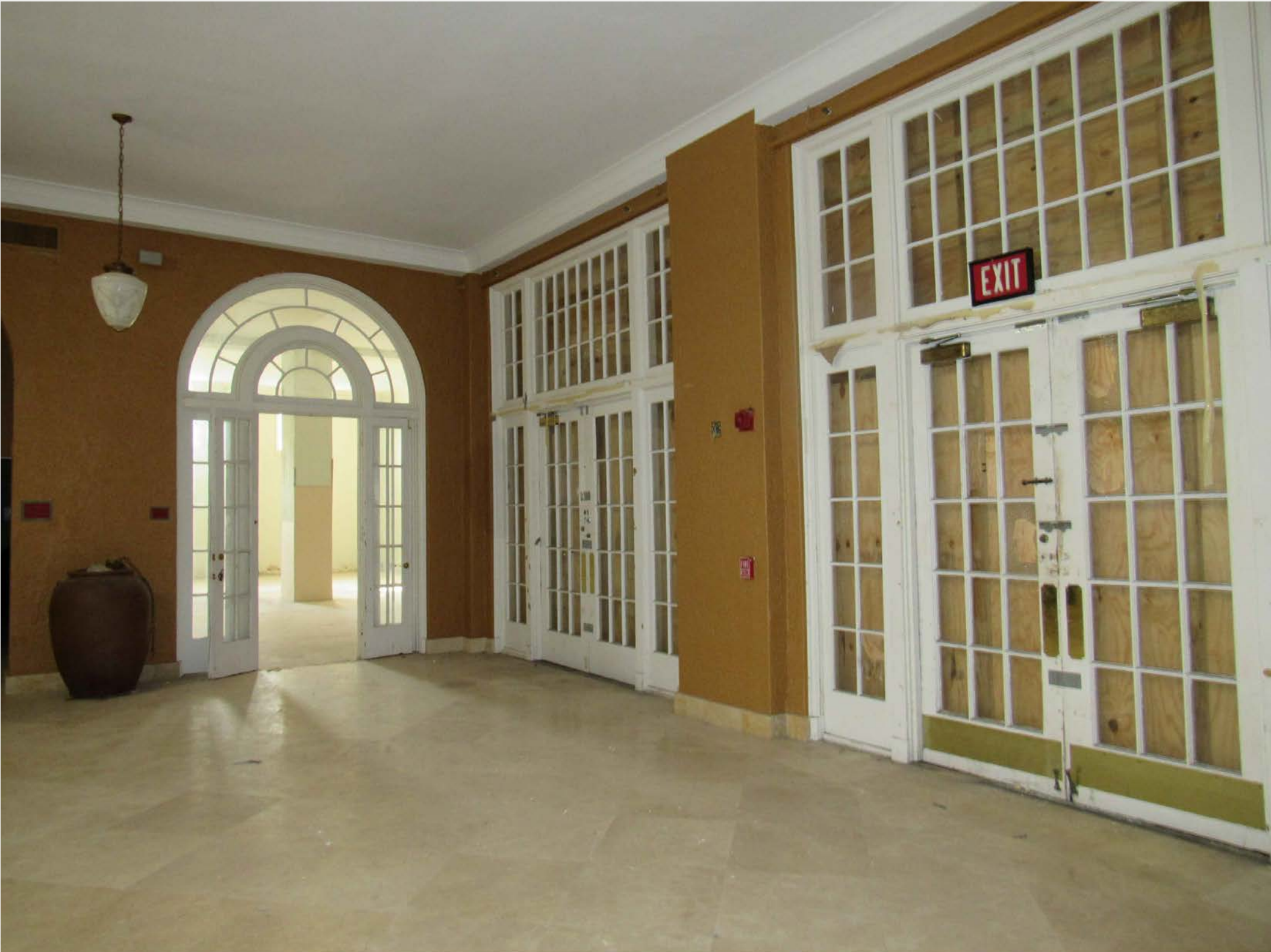
EXISTING FRENCH DOORS TO BE REPLACED WITH NEW DOORS (MULLION CONFIGURATION TO MATCH EXISTING)
