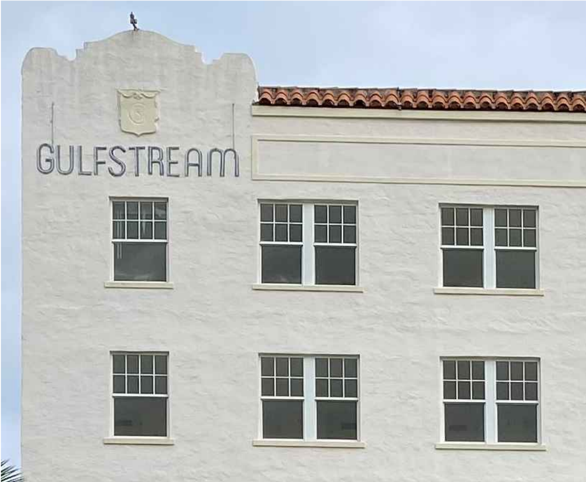
TRIMS CLAY BARREL TILE ROOF GULFSTREAM SHIELD AND SIGNAGE EXISTING WINDOWS TO BE REPLACED WITH NEW WINDOWS (MULLION CONFIGURATION TO MATCH EXISTING)
