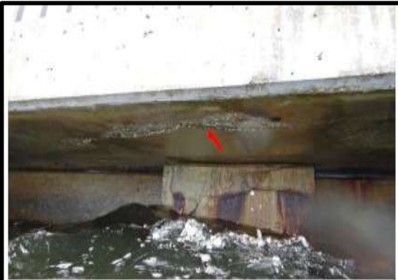
Photo A-39: Delamination on the bottom of the concrete slab at bent 13-a.
