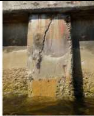
Photo E-55: Deterioration on soldier piles at the casement bulkhead.
