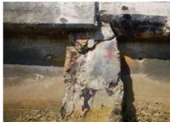
Photo E-56: Deterioration on soldier piles at the casement bulkhead.
