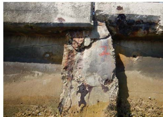
Photo E-56: Deterioration on soldier piles at the easement bulkhead.
