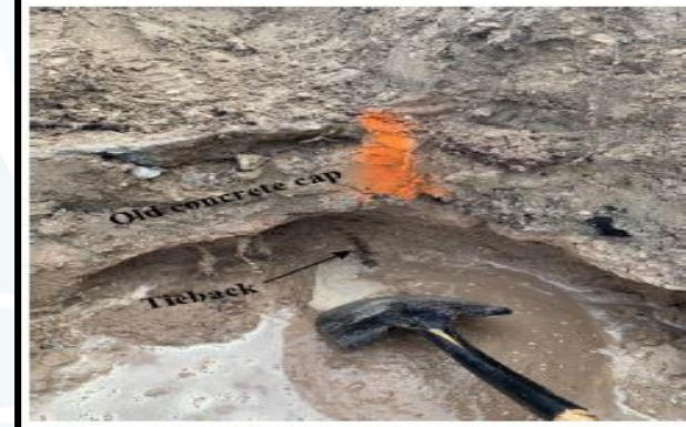
Photo A-70: An old bulkhead was revealed behind the existing bulkhead. A tieback was revealed at station 1+34.
