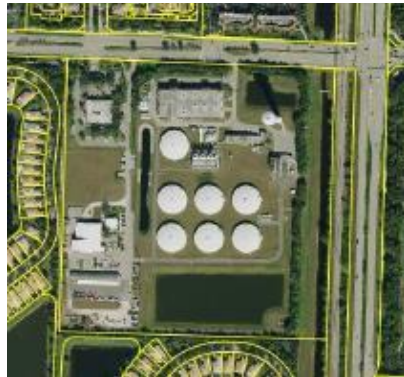
Hood Water Road Plant
