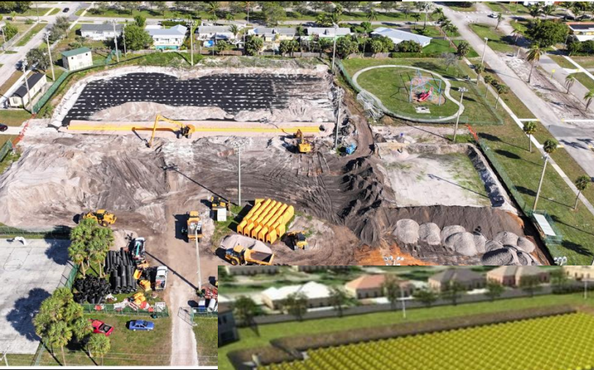
Bostrom Park Project under construction 1/31/25
