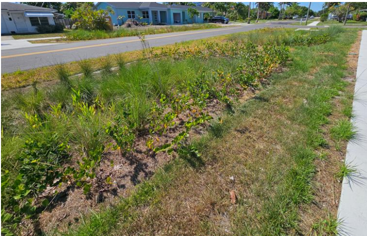
10 th St. Bioswale
