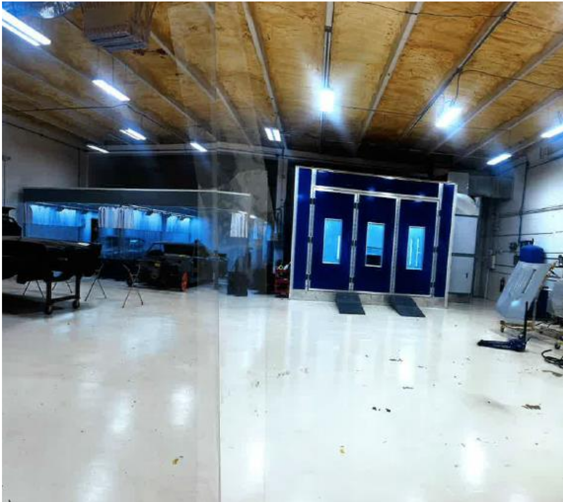
Interior, showing sanding/prep booth on the left and spray booth on the right.
