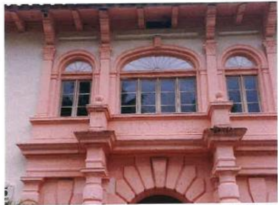
The sections of radius arched windows (above the casement windows) are not impact rated. Building exterior hardening plan is to change these openings to achieve an impact rating.
