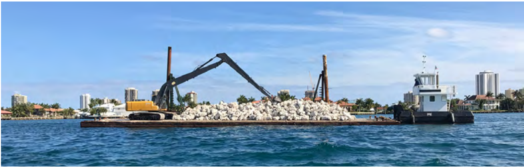
Installing artificial reef at Sugar Sands (Photo credit: PBC-ERM)
