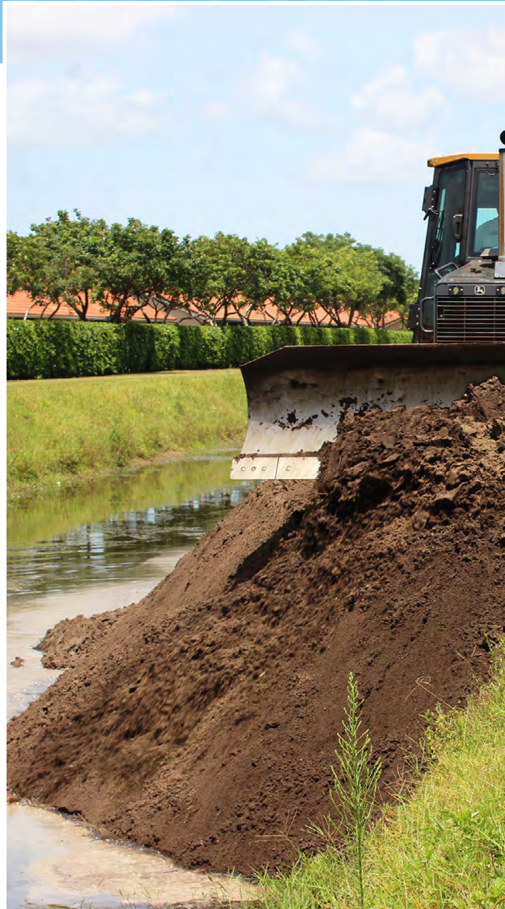
Canal maintenance includes sediment removal to improve flows and functioning of water conveyance canals (Photo credit: Lake Worth Drainage District)
