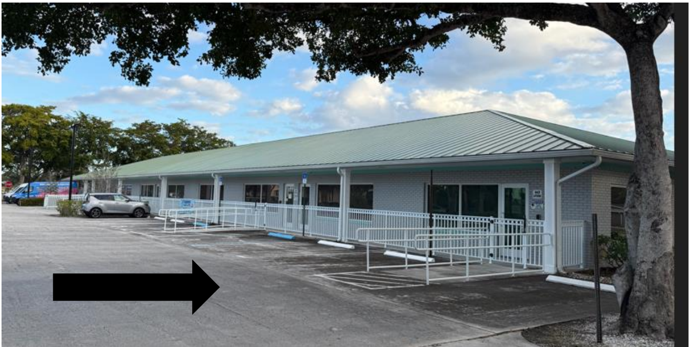
South End of Building – Proposed Location
