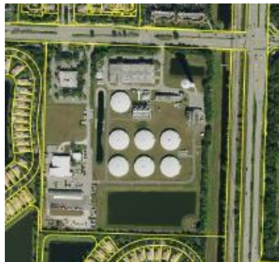
Hood Water Road Plant
