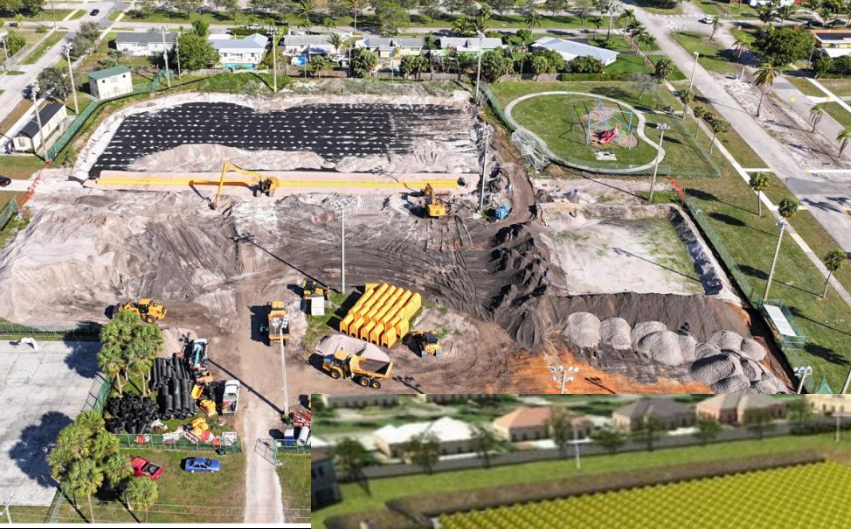
Bostrom Park Project under construction 1/31/25
