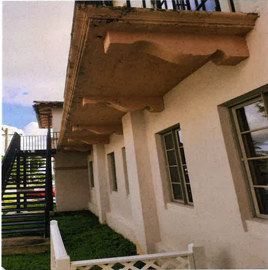
WEST SIDE BALCONY with CONCRETE CANTILEVERED SUPPORT BEAMS
