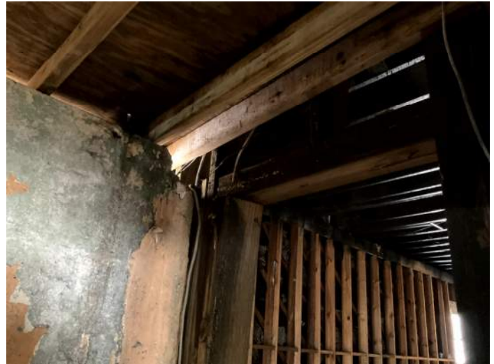
Broken top of bearing wall, joist not supported PHOTO NO. 20230710_180056949
