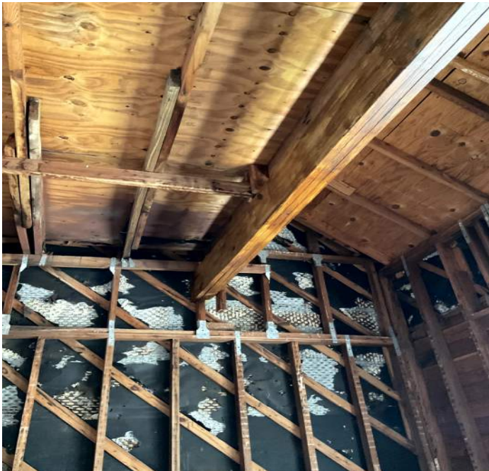
Unconventional top of wall framing PHOTO NO. 20230710_182333863
