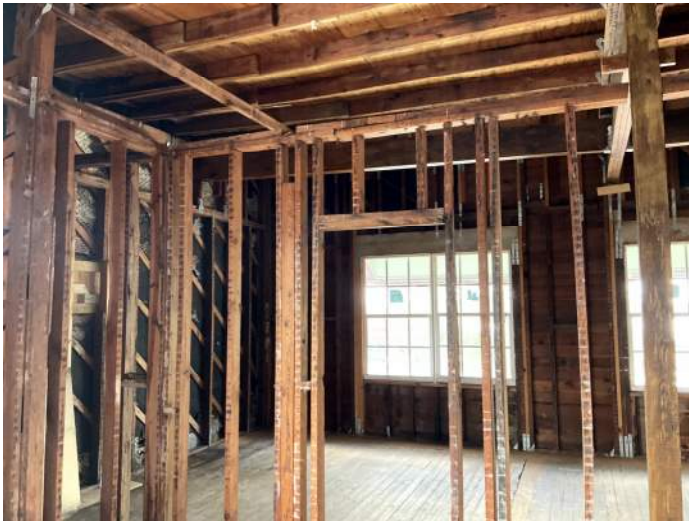
2 nd Floor interior wall framing PHOTO NO. 20230710_182257563
