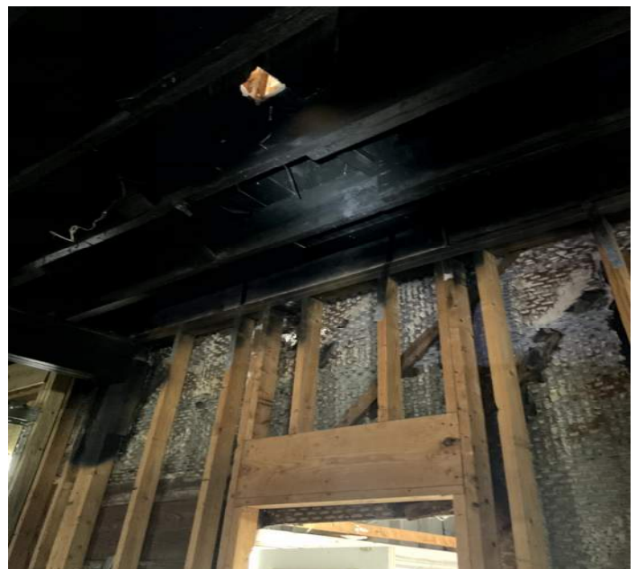
Original rear wall framing, exposed stucco lath, unfinished PHOTO NO. 20230710_180851909
