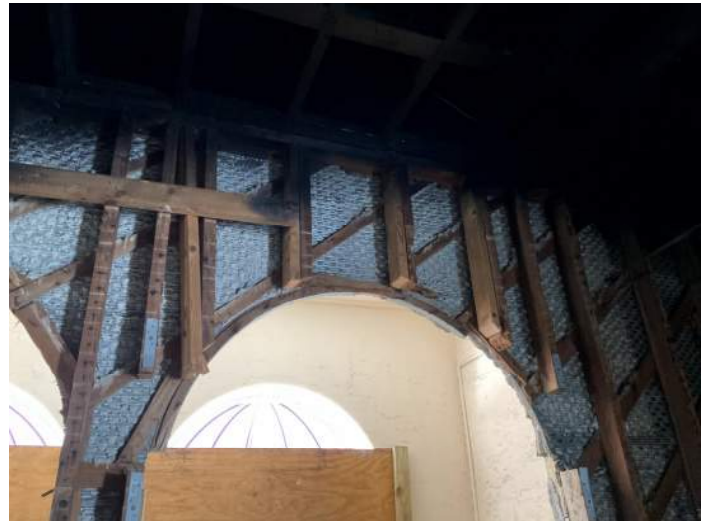
Missing header over arched openings PHOTO NO. 20230710_181658453
