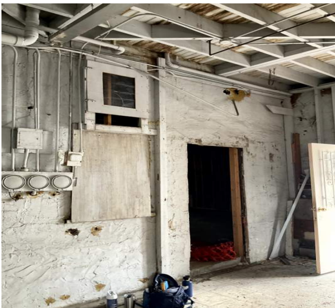
Original back wall, water damage, unfastened stucco finished PHOTO NO. 20230710_180139050
