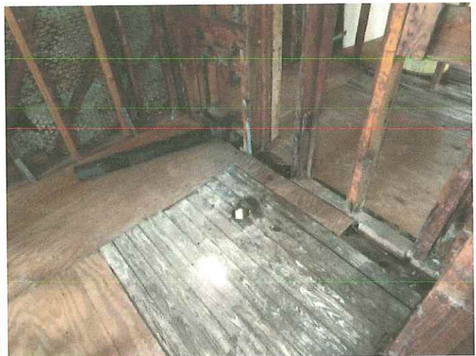
Discontinuous floor deck sheathing PHOTO NO. IMG_8011
