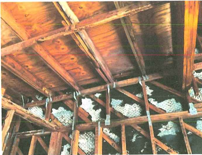
Spliced roof joist framing at bearing ends PHOTO NO. 20230710_182352450
