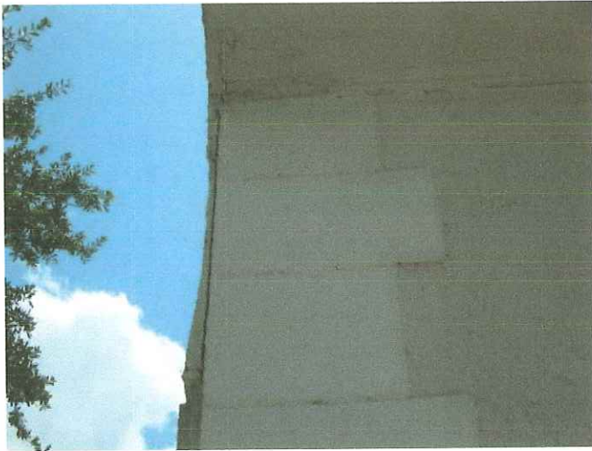
Finish separation PHOTO NO. IMG_7919
