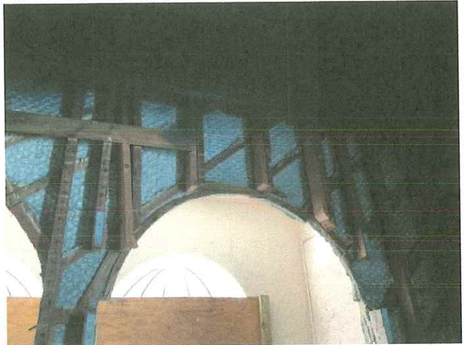
Missing header over arched openings PHOTO NO. 20230710_181658453
