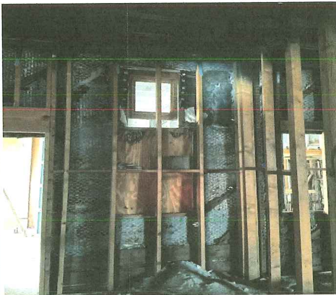
Original rear wall framing, exposed stucco lath, unfinished PHOTO NO. 20230710_180812979
