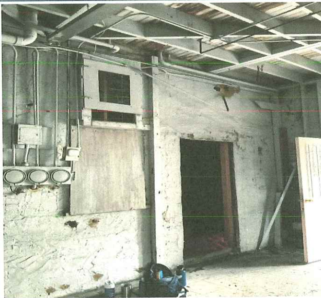
Original back wall, water damage, unfastened stucco finished PHOTO NO. 20230710_180139050
