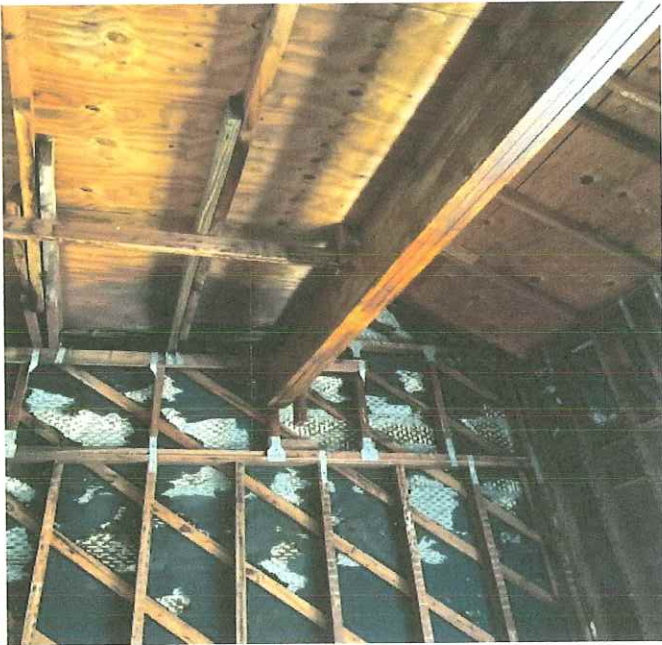
Unconventional top of wall framing PHOTO NO. 20230710_182333863
