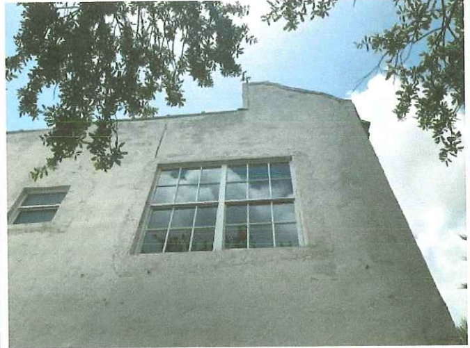
Stucco repair transition around window PHOTO NO. 20230710_175305873
