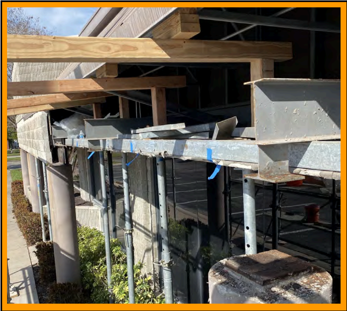
An extensive shoring system was installed to replace and repair the I-Beam lintels.
