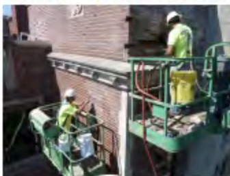
Tuckpointing & Brick Repairs
