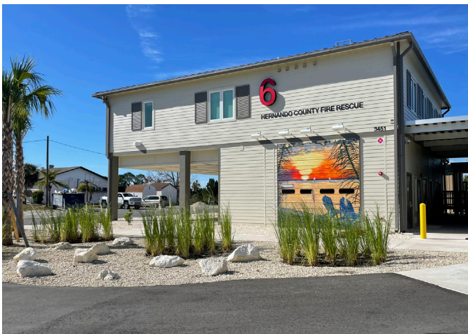
Hernando County Fire Station No. 6
