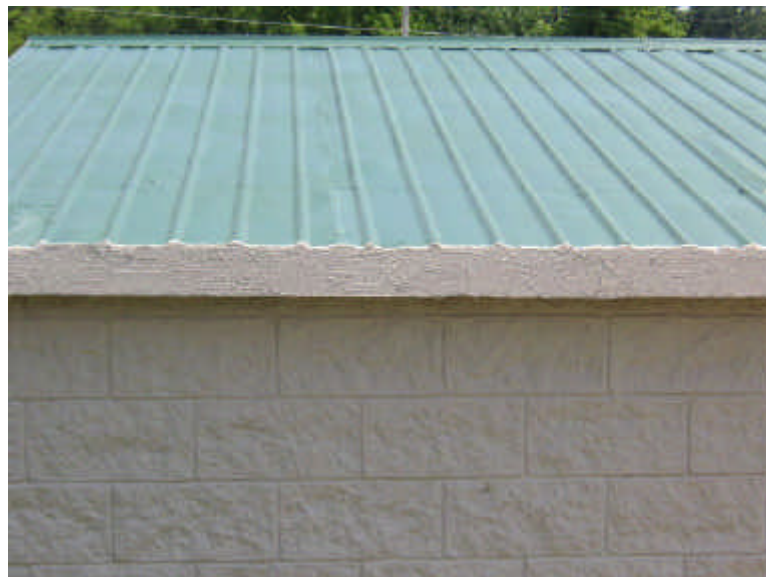
ROOF DETAIL SIMULATED RAISED SEAM METAL
