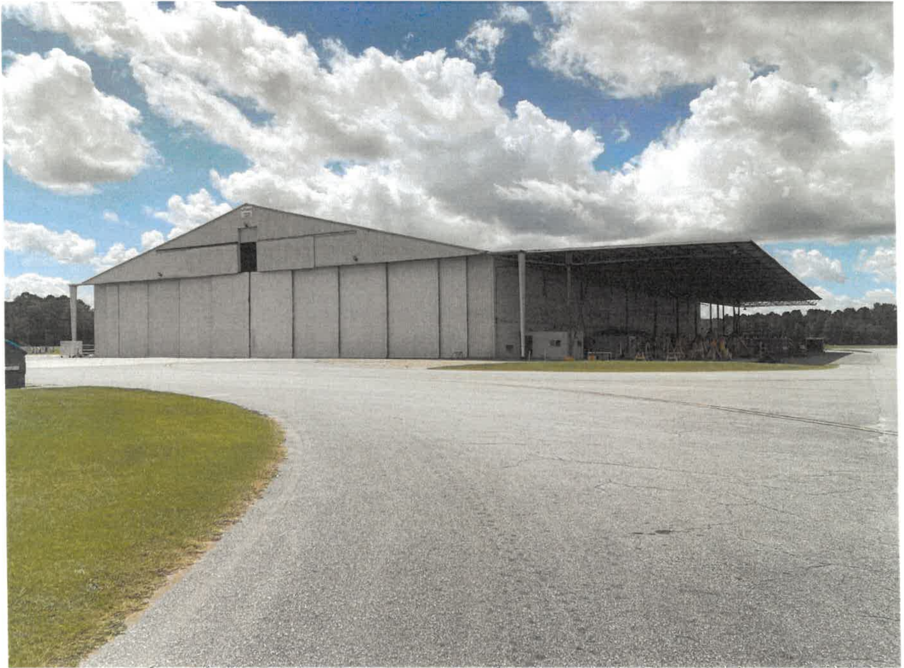
Hangar 4 – North Side
