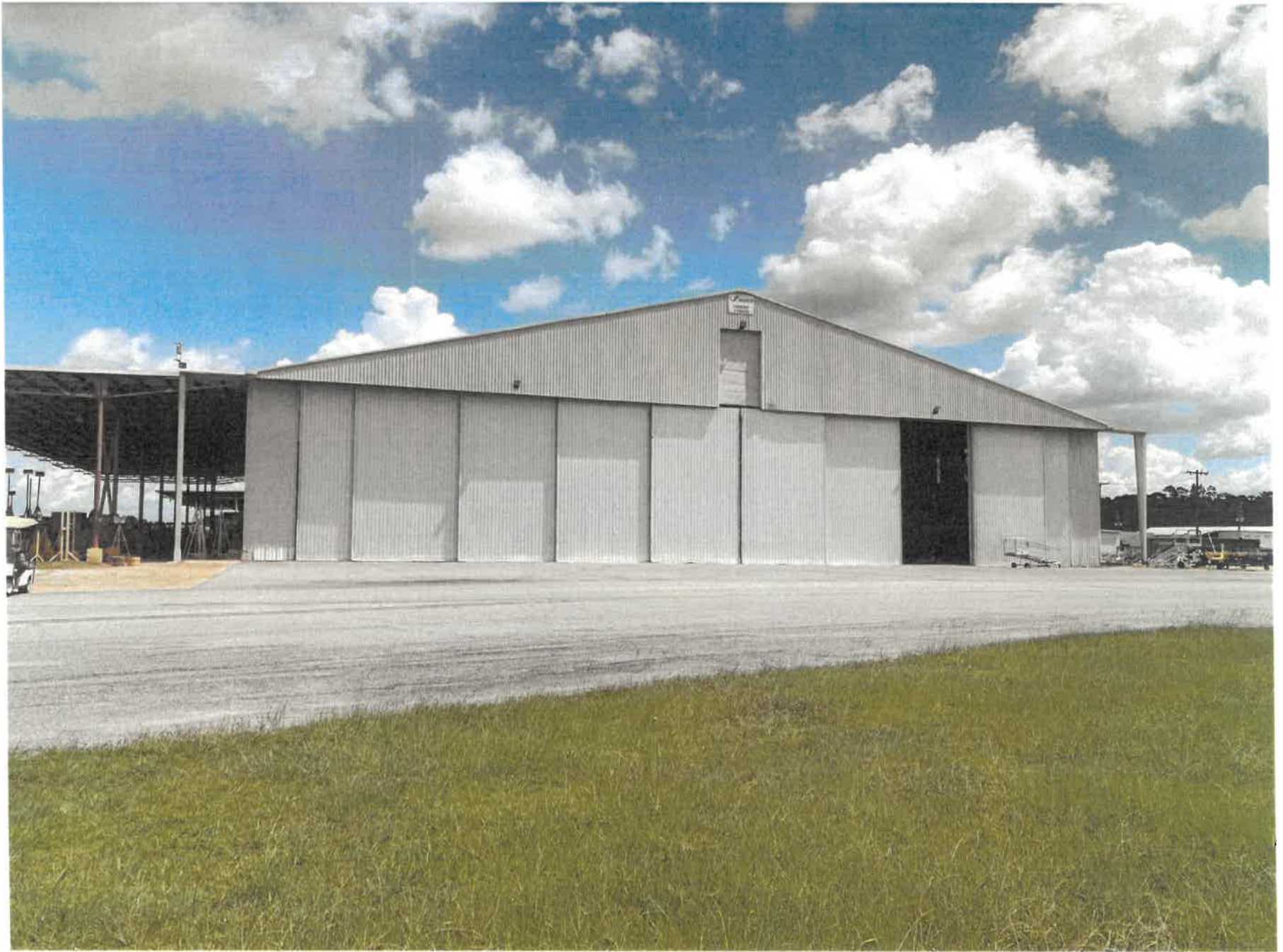
Hangar 4 – South Side
