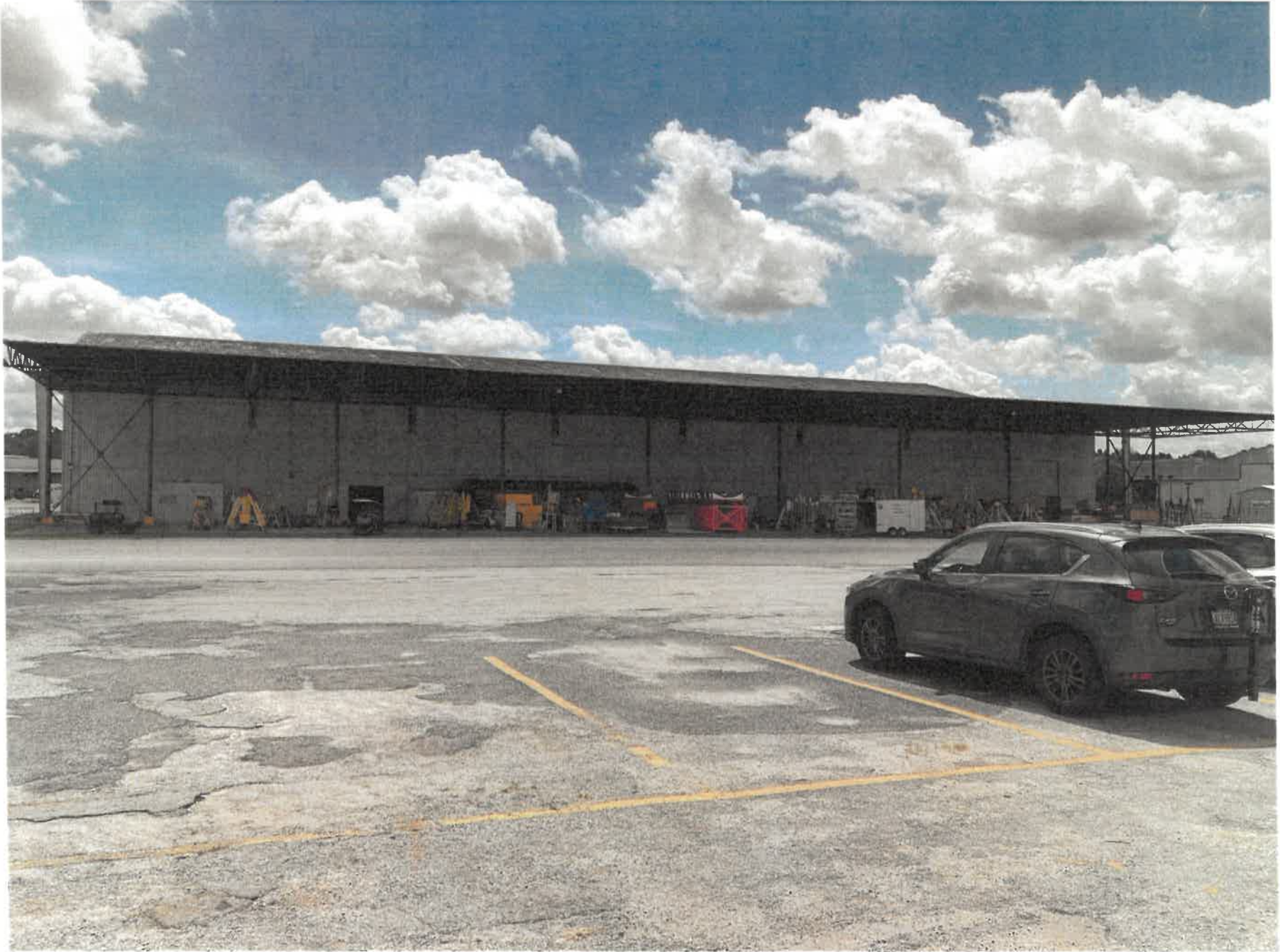
Hangar 4 – West Side
