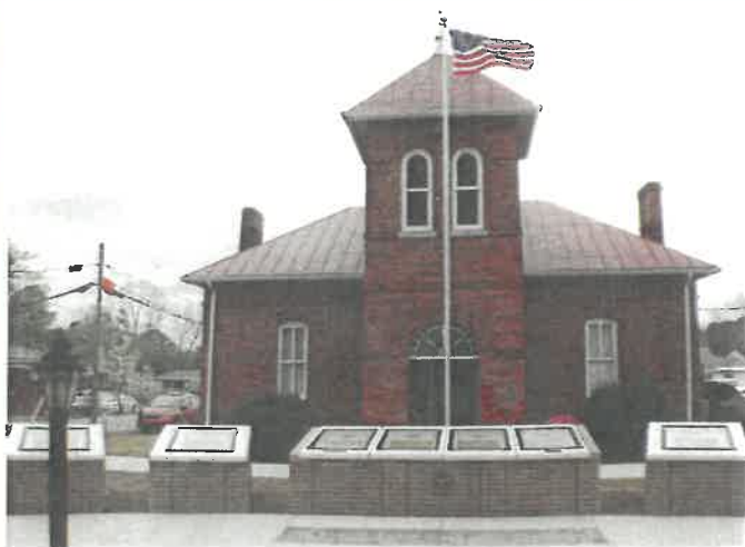
Halifax County, Halifax, North Carolina Local Brick with Cast Stone Cap and Chambers With Halifax Resolves on the far left. Dedicated April 12, 2019
