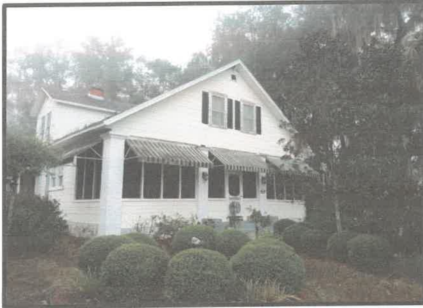
Current Front Façade
