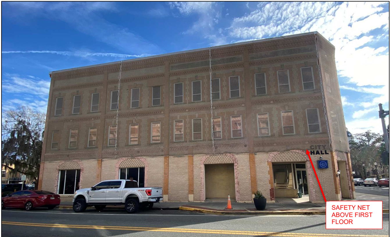
Photo 1: West Building Face
