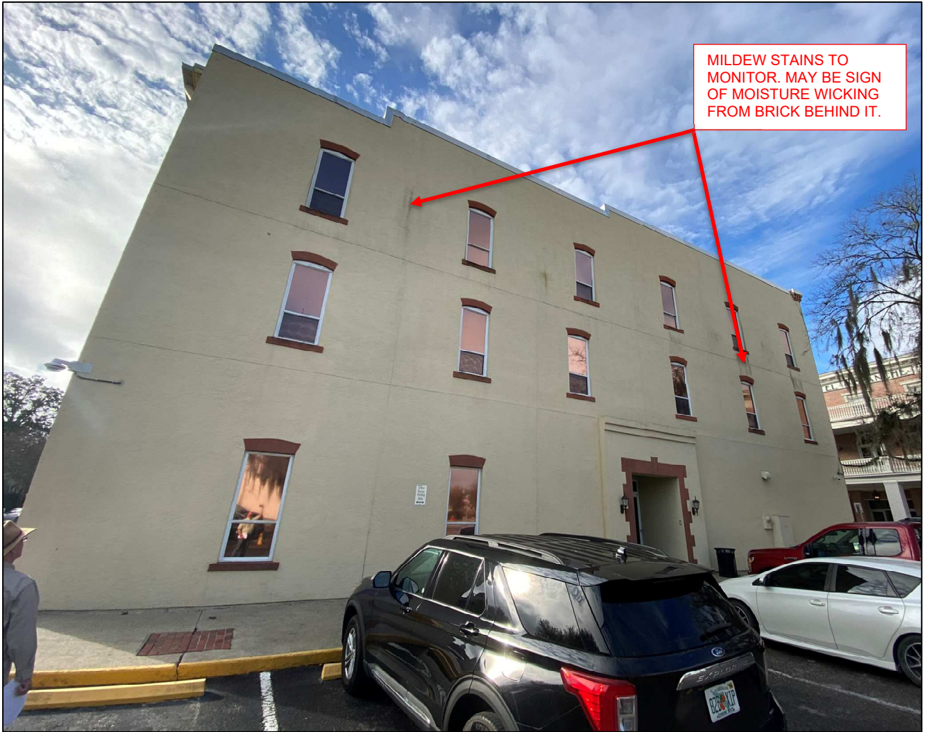
Photo 3: North Building Face
