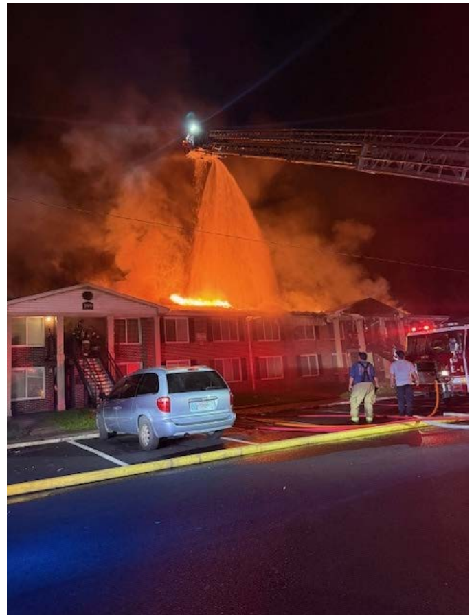
Cedar Park Structure Fire
