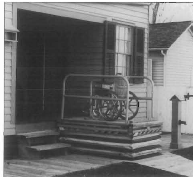
An accordion-type platform lift that retracts to ground level when not in use has been installed to make this historic house accessible.
