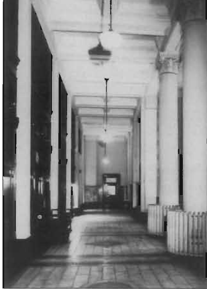
The visible features of historic mechanical systems, such as heating, lighting, and plumbing, may sometimes help define the overall character of an interior.
