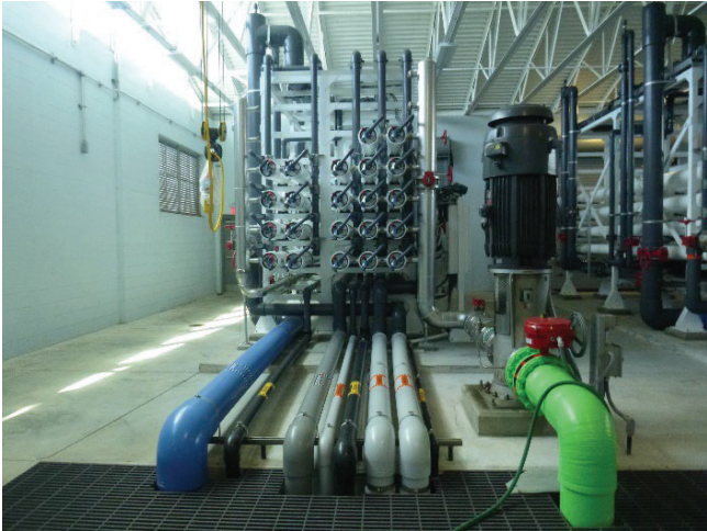
Photo 1: View of first train in RO system.
