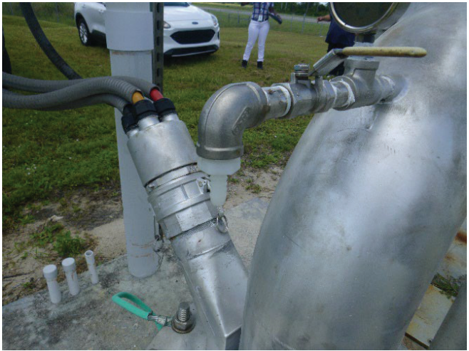
Photo 22: View of plug on raw sample tap.
