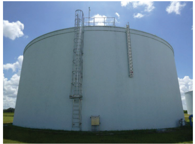
Photo 14: View of ground storage tank.
