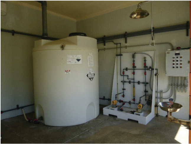
Photo 7: View of chlorine tank 2.
