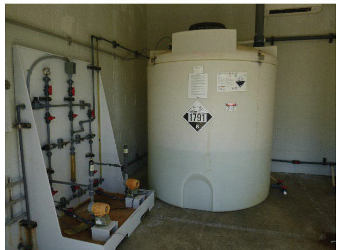
Photo 6: View of chlorine tank 1.
