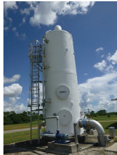
Photo 4: View of degasifier.
