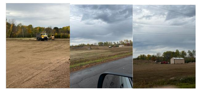
Yard Waste site gravel install (2957 tons of material in place)
