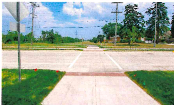
SOUTH 68TH STREET CONCRETE REPLACEMENT GREENFIELD, WI
